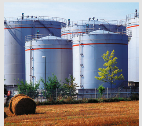
Industrial steel constructions
